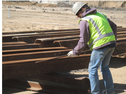
REMOVE DEBRIS BY AIR AFTER CLEANING INTERLOCKS
