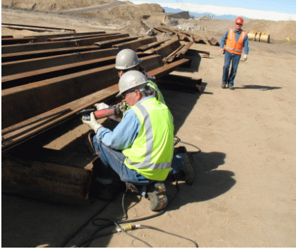
CLEANING INTERLOCKS WITH DRILL MOUNTED WIRE BRUSH
