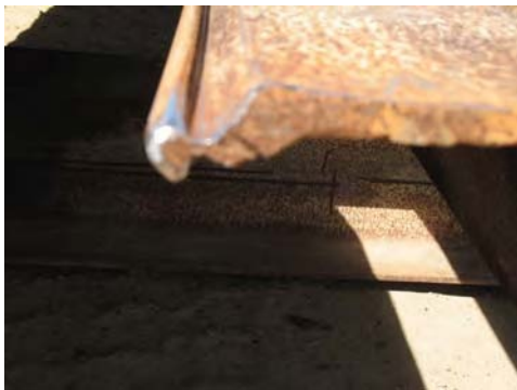
“Ball” of PZ piles - grind off any rough edges of the ball before driving. Rough edges could gouge A-30 from the socket
