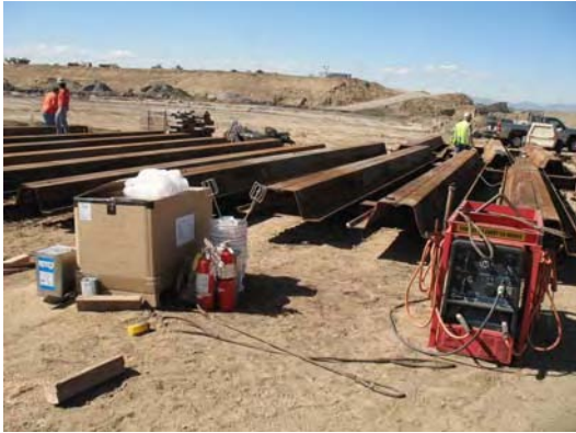
Place piles on parallel level H- Beams
